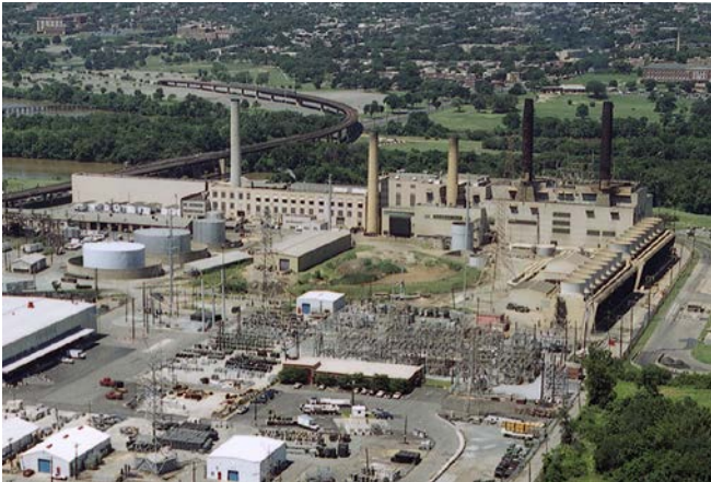
Benning Power Plant before demolition
