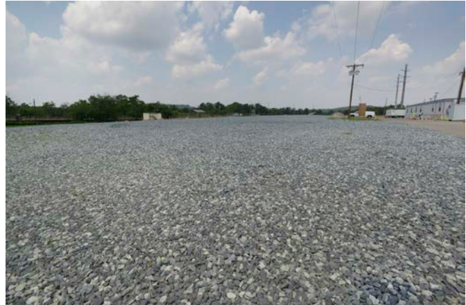
Benning site after demolition completed (looking north from near Benning Road)
